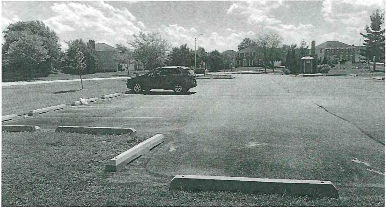
Figure 3a: Parking Lot
