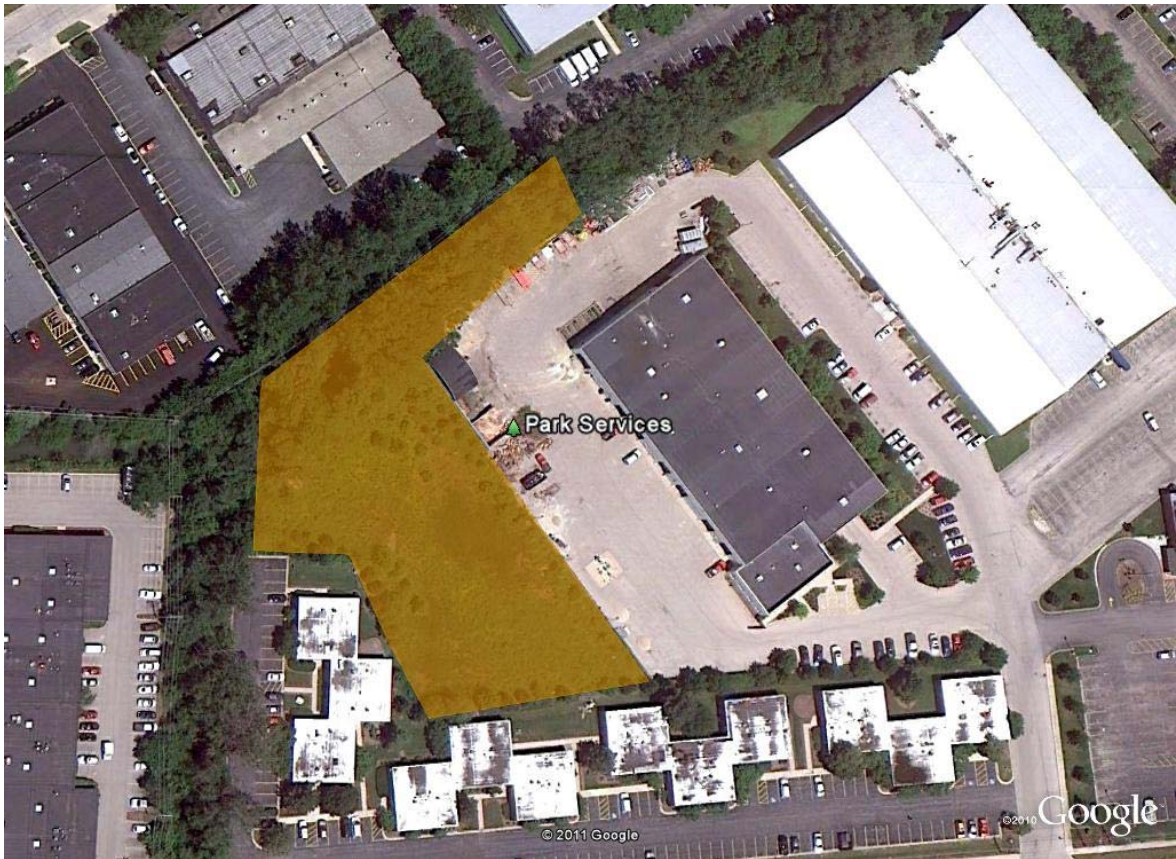
Park Services is the 4.3 acre maintenance facility and contains 1.55 acres of naturalized retention.
